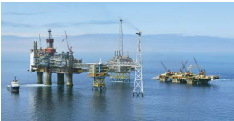
Fire water and seawater lift pumps at Sleipner field. Photo: Courtesy of Statoil.
