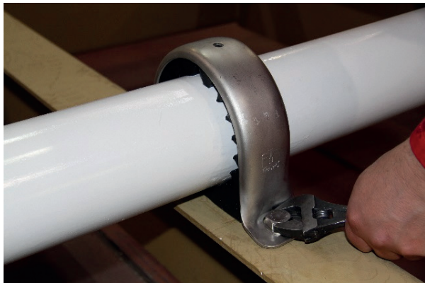
Tighten the bolts
