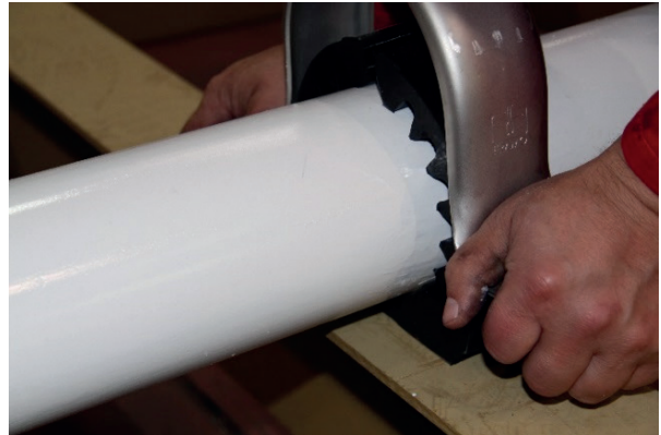
Re-install the pipe clamp steel body.
