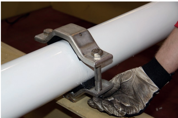
Re-install the upper clamp body. Tighten the bolts.
