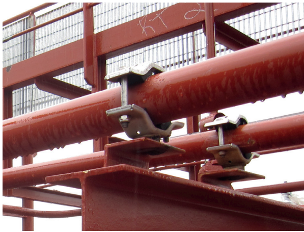
Pipe clamp type delivered before 2007
