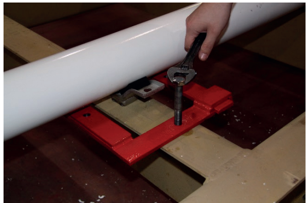
Lift the pipe off the rubber element by turning the bolts.
