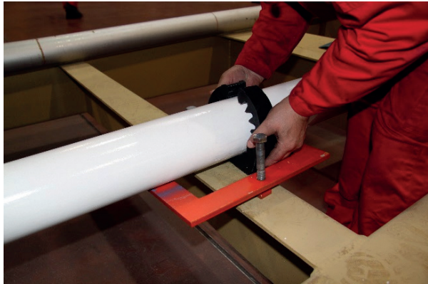
Let the paint dry. Check the flexible rubber element for wear/damages, and renew if necessary before re-installing.
