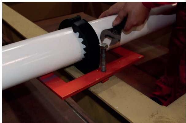
Place the lifting tool underneath the pipe, and lift the pipe off the rubber element by turning the bolts.
