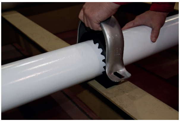
Remove the bolts and lift of the steel body
