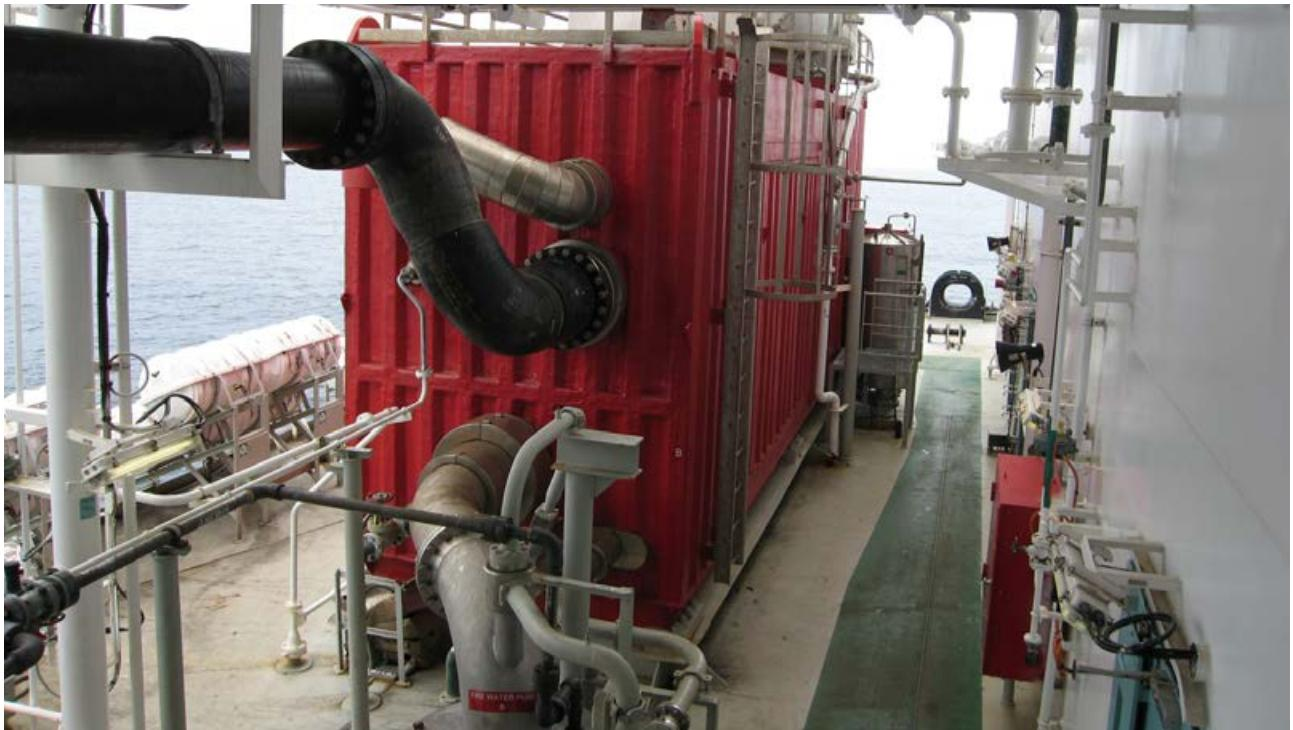
A fire detection and extinguisher system is installed to detect and extinguish a potential fire inside the container. The type of extinguisher system can be water mist, inergen or CO<sub>2</sub>.
