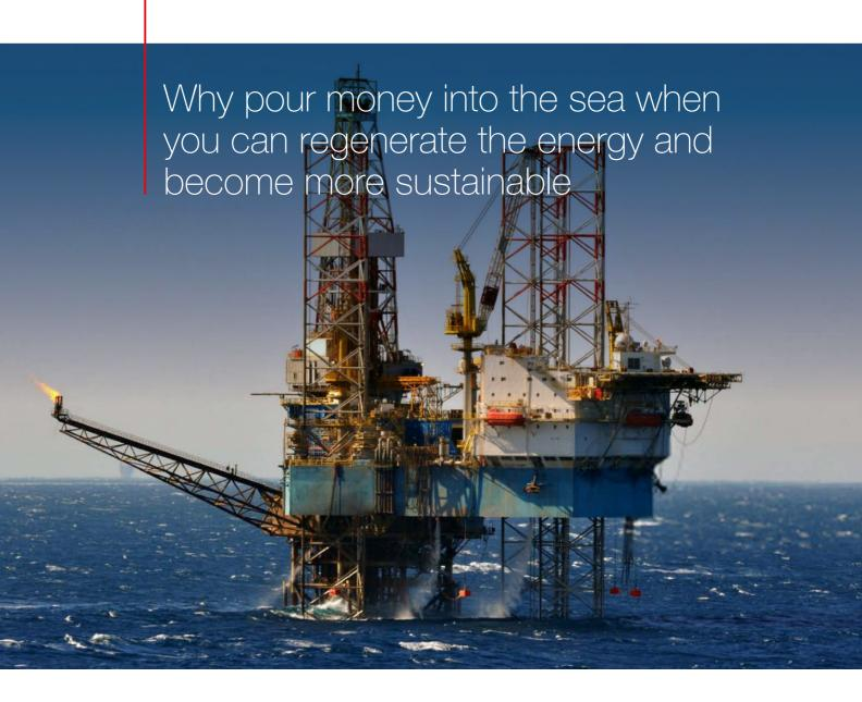
During offshore oil production, a massive amount of seawater is pumped up from the sea to deck level at great energy costs. Once the sea water has served its purpose of cooling down the oil, it is simply dumped back into the sea. Substantial energy goes to waste.
