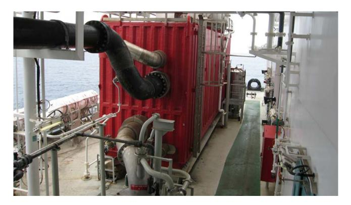
A fire detection and extinguisher system is installed to detect and extinguish a potential fire inside the container. The type of extinguisher system can be water mist, inergen or  $CO_2$ .
