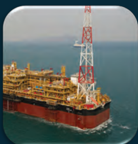
Offshore pumping system
