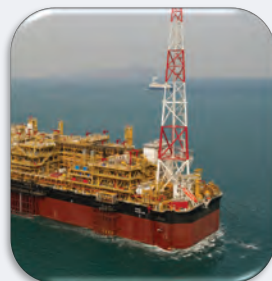
Offshore pumping system
